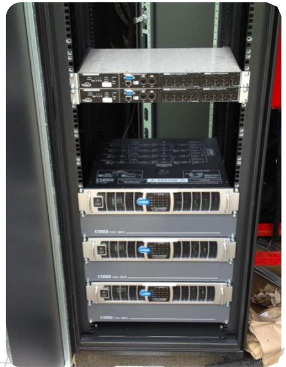
Area rack detail during mounting : Cloud amplifiers connected to EtherSound through AuviTran AudioToolBox
